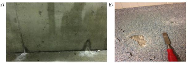
Fig. 1. Examples of issues caused by leaking groundwater through concrete floors in underground structures including: a – unsightly leaks, collection of water and long-term durability concerns; b – poor performance of floor coatings or covering
